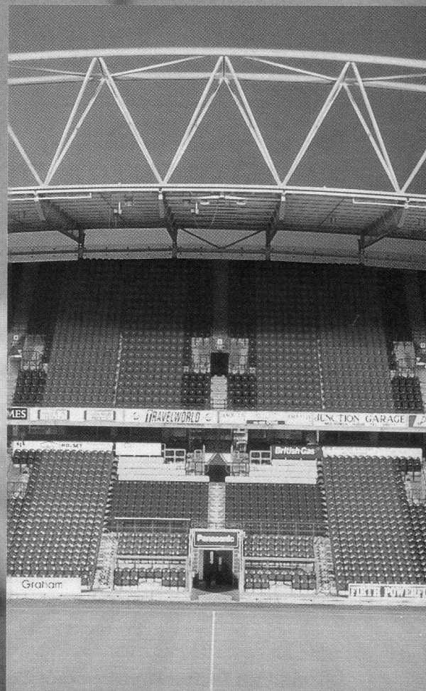
The Lawrence Batley Stand at The Alired McAlpine Stadium
